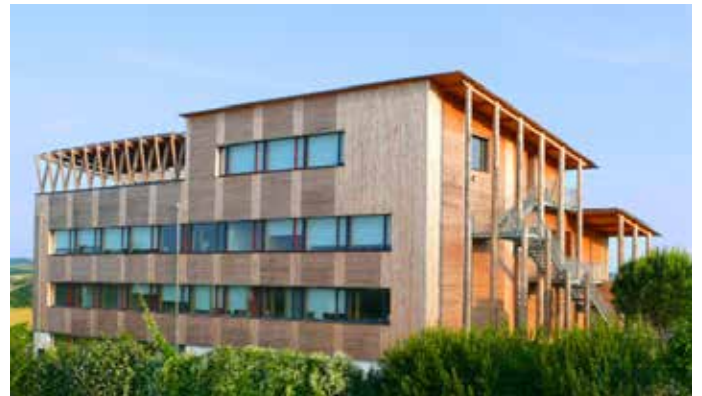
ECOCERT headquarters based in the south of France is an Energy Plus building: wooden framework, thermal insulation with straw, low energy consumption, solar panels...
